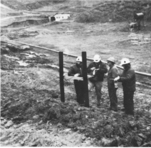
Fig 1 Lagoon embankment showing three acoustical waveguide rods (3/8-in o d reinforcing rods) from embankment (left) to monitoring station (center) View is of downstream side of embankment
