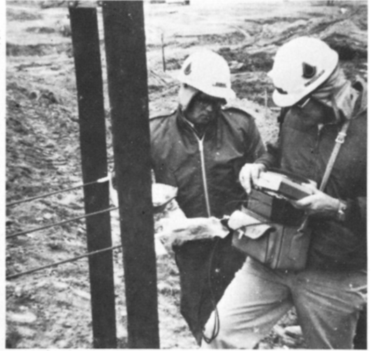
Fig 1 Lagoon embankment showing three acoustical waveguide rods (3/8-in o d reinforcing rods) from embankment (left) to monitoring station (center) View is of downstream side of embankment
